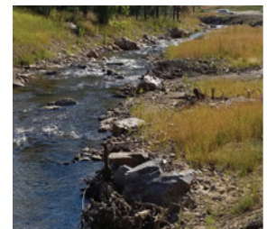
Riparian regeneration after one season of growth and root wad revetment with habitat wood
