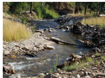
Riparian regeneration after one season of growth and root wad revetment with habitat wood
