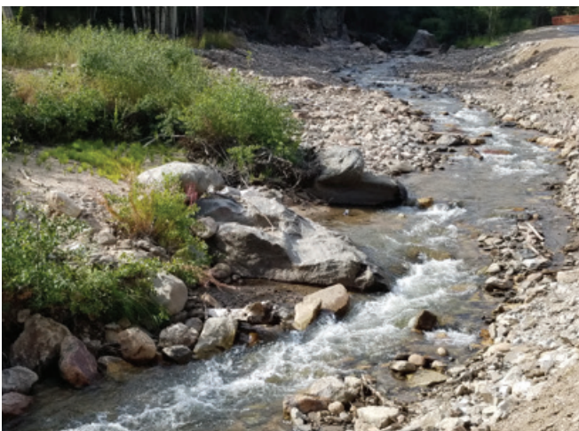
Floodplain grading and boulder placement.
